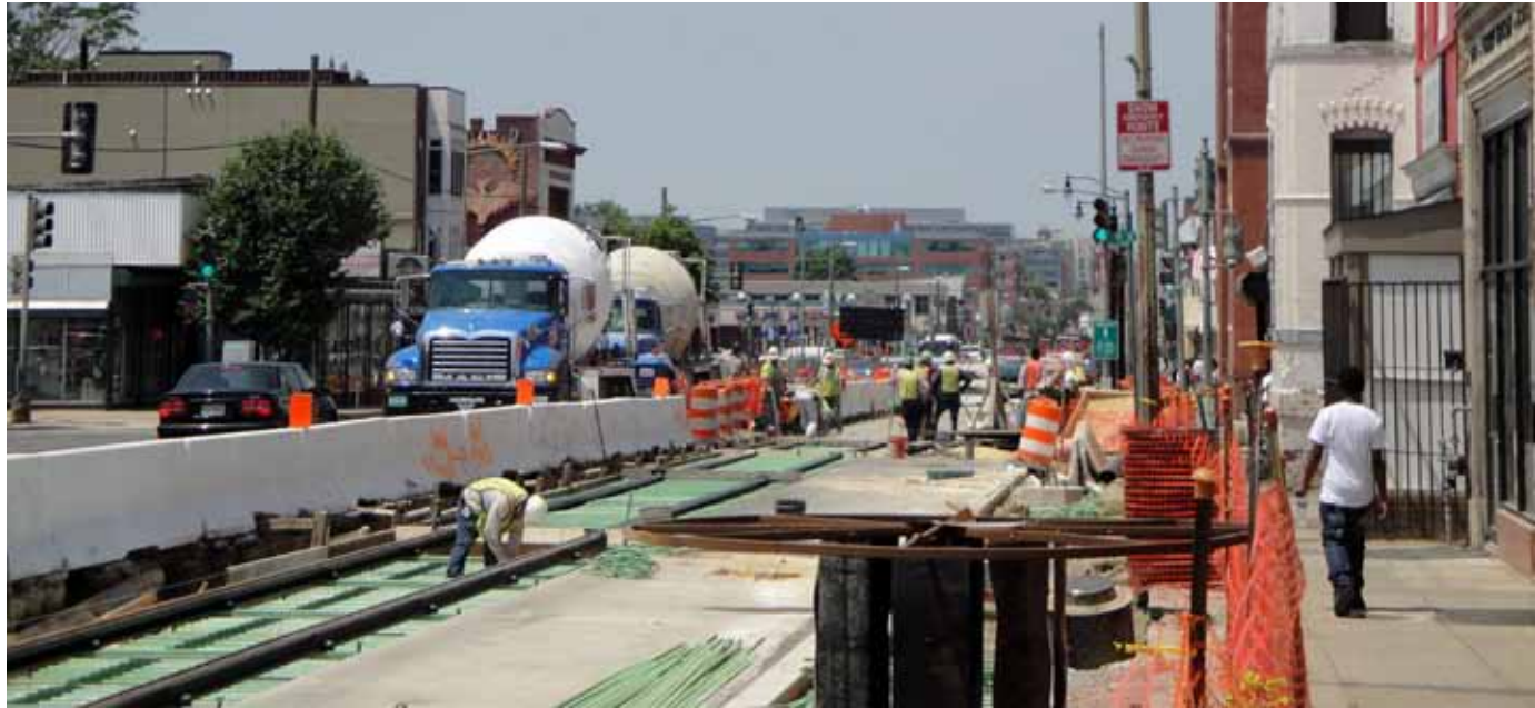
Construction of the H Street/Benning Road NE streetcar segment, August 2010
