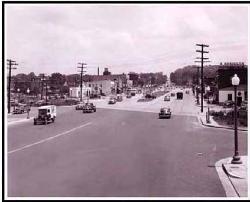
Photograph courtesy of DDOT.
