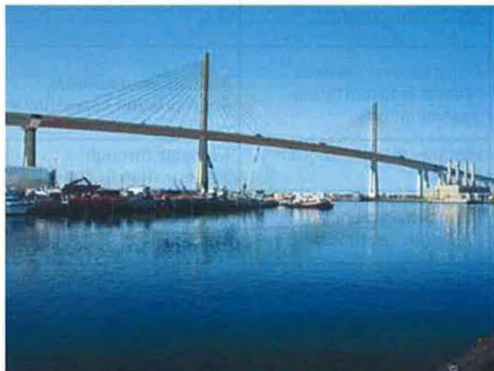
Port of Long Beach, CA, Gerald Desmond Bridge Replacement
