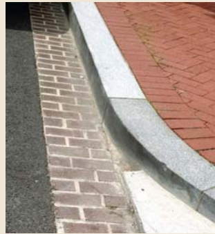
Granite Curb/Brick Gutter
