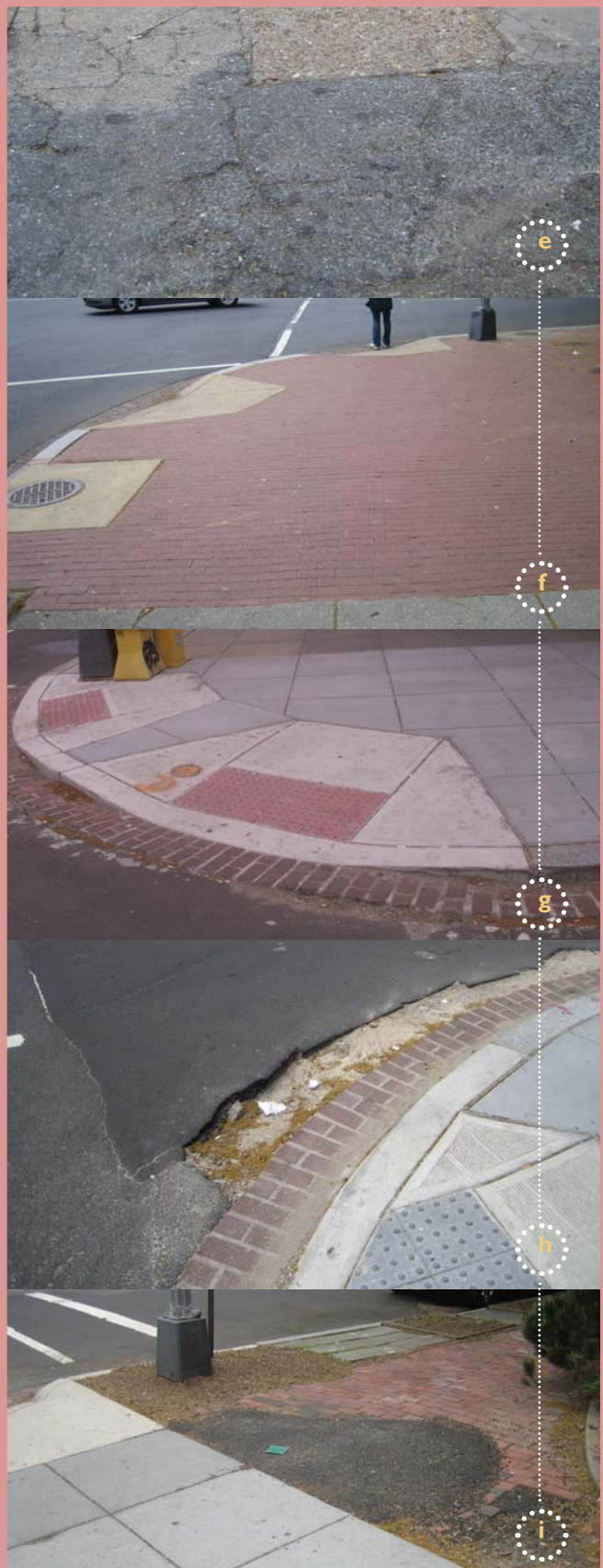
Patchwork of Sidewalk Materials
