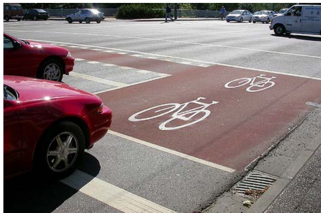
Figure 5.9 - Vancouver Precedent: Bike Waiting Area at an Intersection
