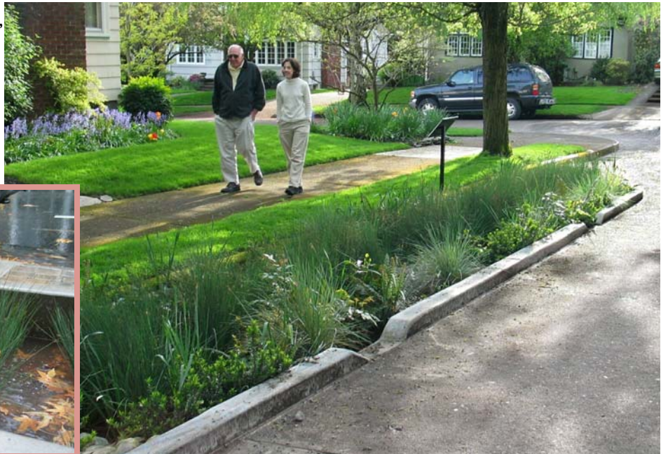
Figure 6.27 - Siskiyou Street Portland, Oregon - Landscaped Stormwater Curb Extension (ASLA Photo)
